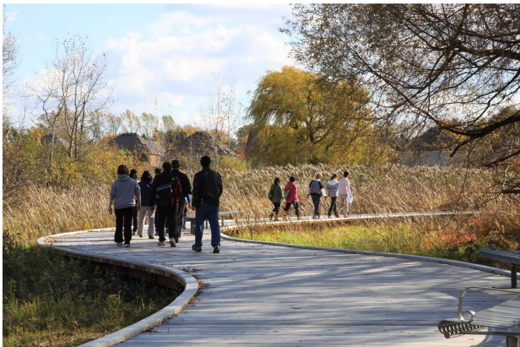
The boardwalks built on helical piers tread lightly through the wetlands
